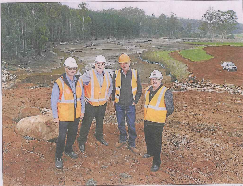
RELIABILITY: Checking progress on the Dial Blythe Irrigation Scheme dam are Shaw Contracting chief executive Hugh Maslin, Braddon MHR Brett Whiteley, Tasmanian Irrigation chief executive Chris Oldfield and Bob Dunk, of pipeline manufacturer Zest. Picture: Grant Wells.
