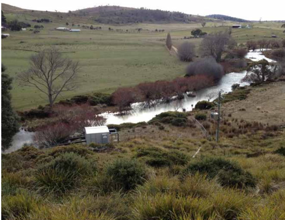
Shannon River Pump Station (SRPS) Site
