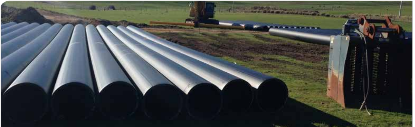
First deliveries to site of DN630 HDPE pipe
