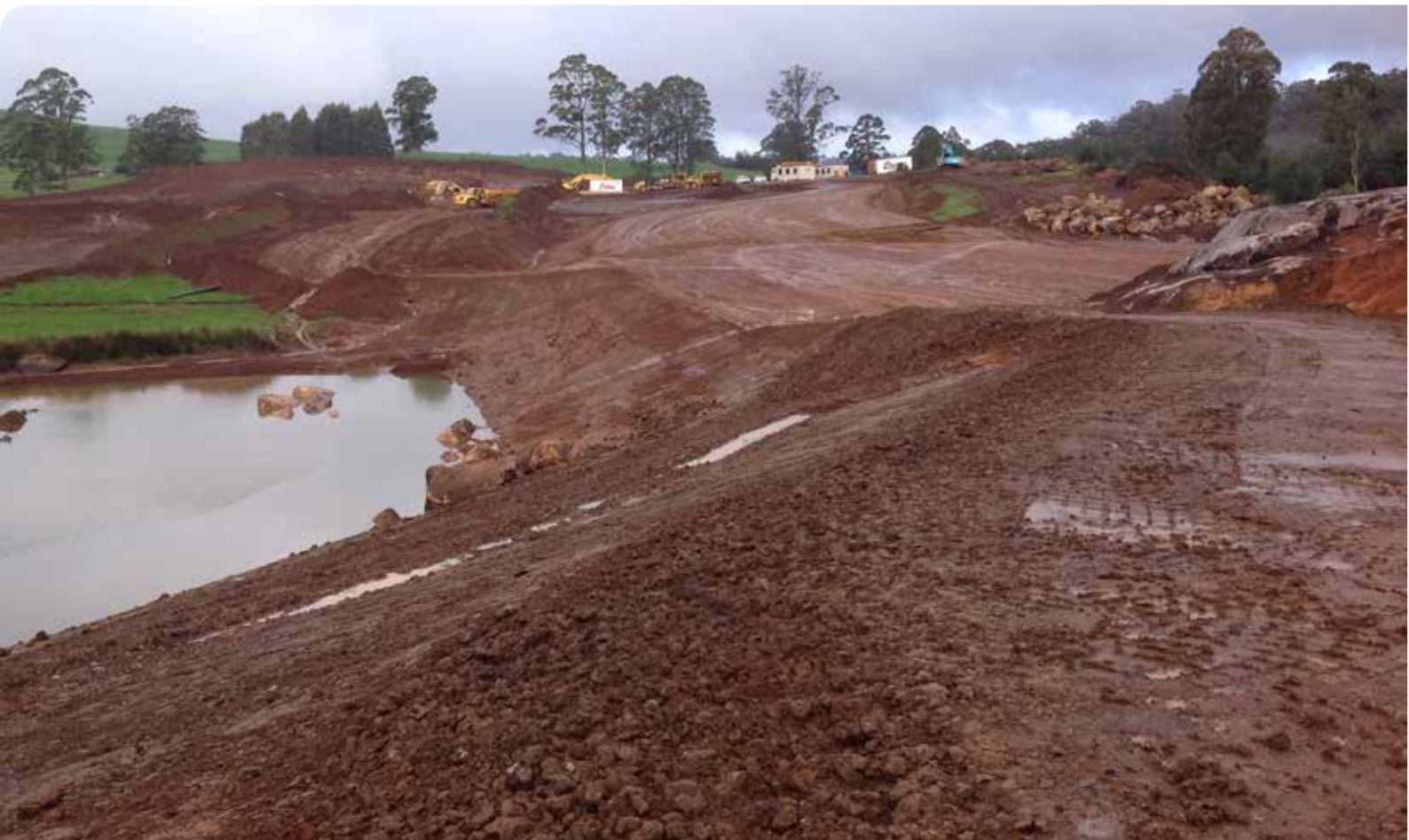
Figure 1: Wall construction 15 July 2014
