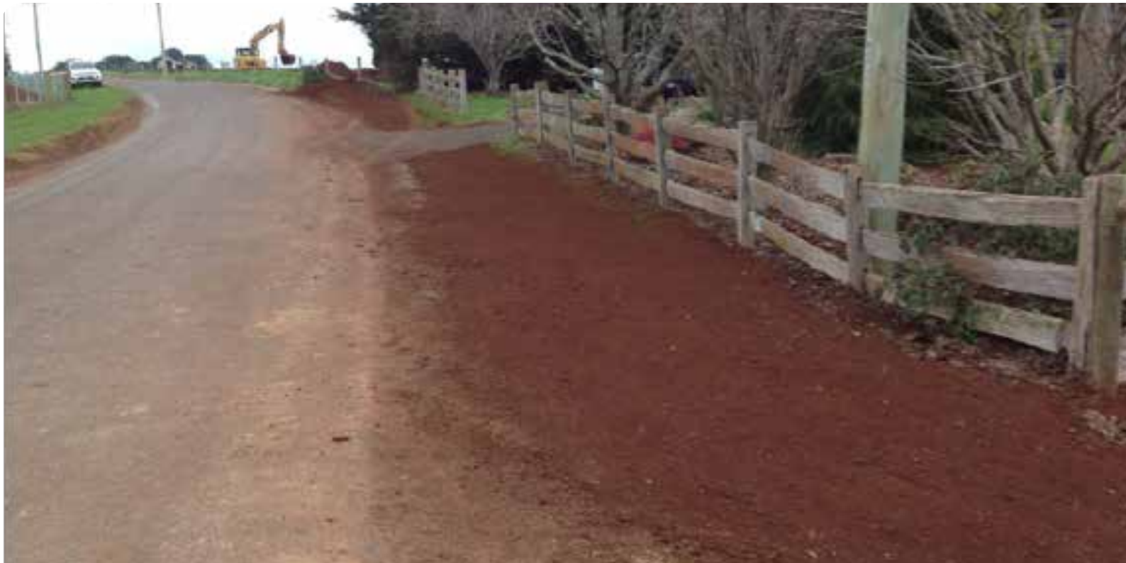
Figure 4: Nature strip rehabilitation after pipe install, Curprona Road
