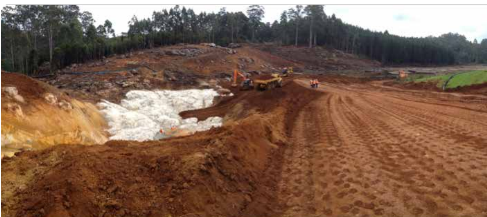
Figure 7: Backfilling the keyway
