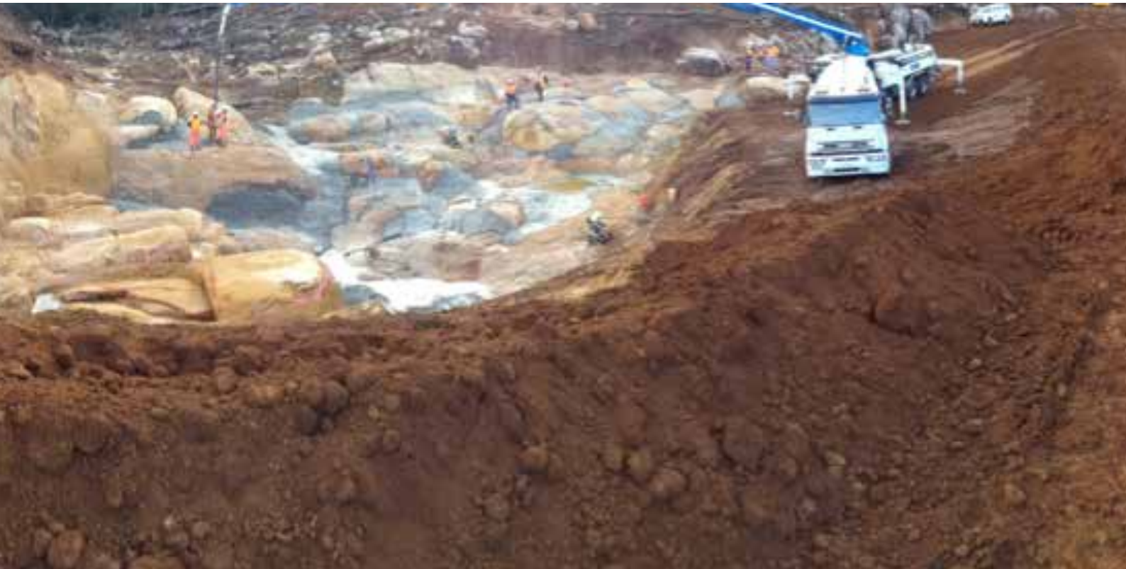
Figure 6: Keyway nearly ready for back fill
