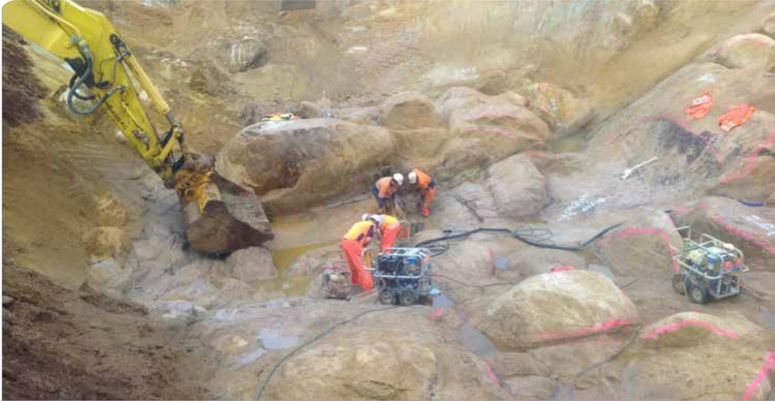
Figure 5: Cleaning the keyway
