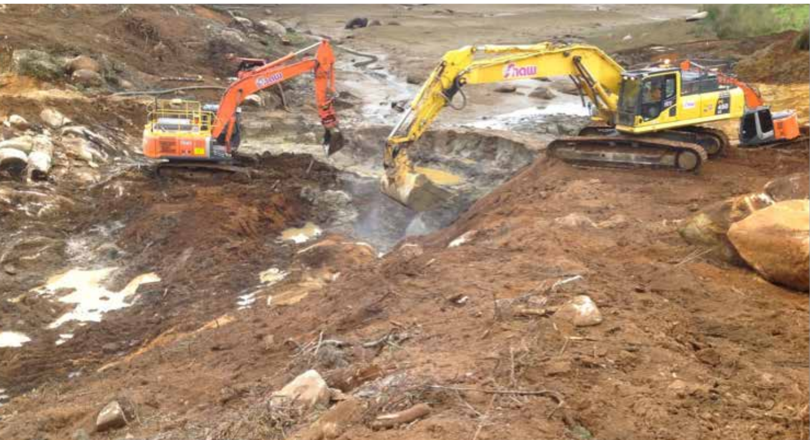
Figure 4: Digging the keyway
