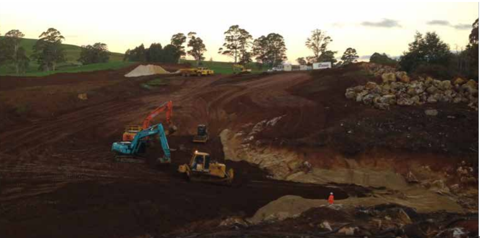
Figure 8: Placing the sand blanket filter downstream of the keyway
