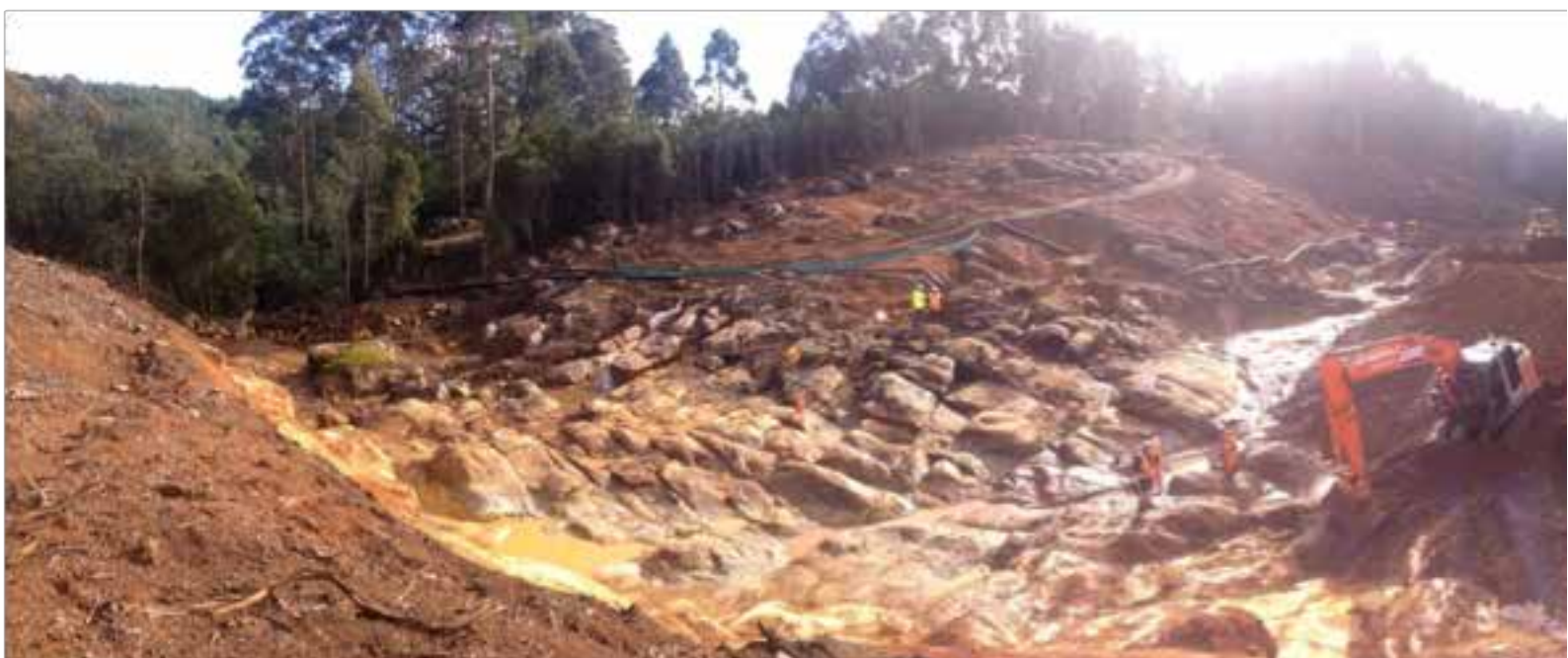
Figure 2: Cleaning of the downstream footprint and placement of the core 23 May 2014
