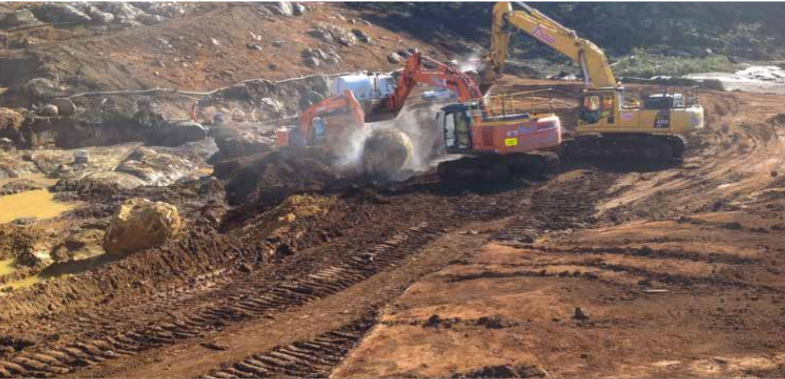
Figure 3: Removing rocks from the keyway
