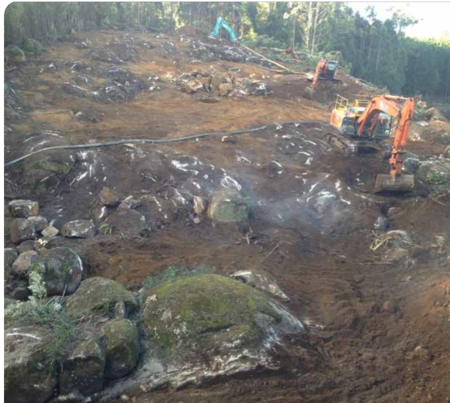
Figure 1: Clearing the embankment 14 April 2014
