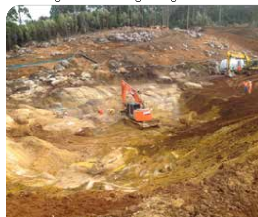
Keyway cleaning during construction of the dam
