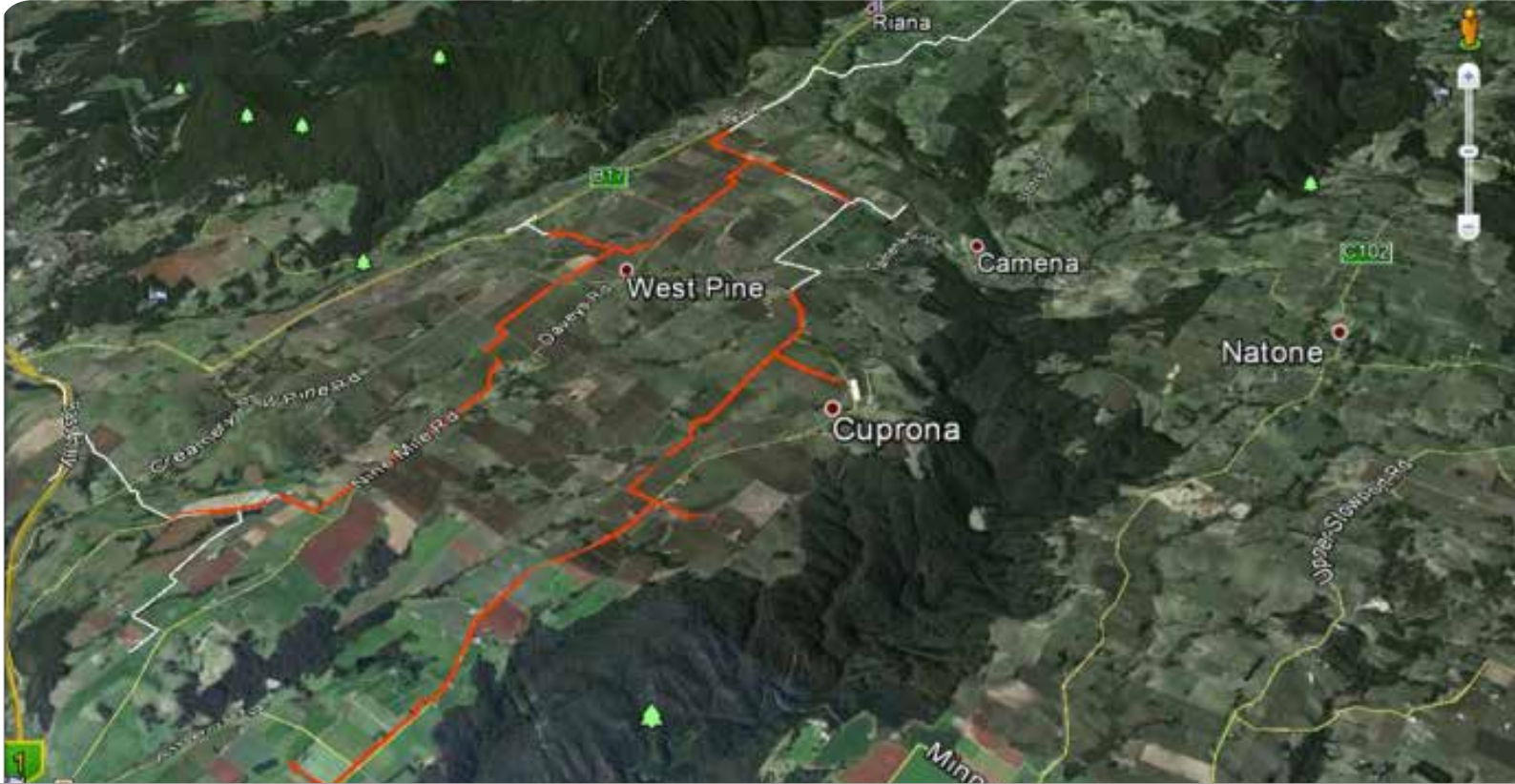
Figure 5: Pipeline installation progress
