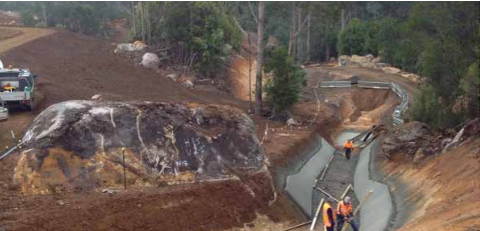
Figure 3: Spillway concreting works
