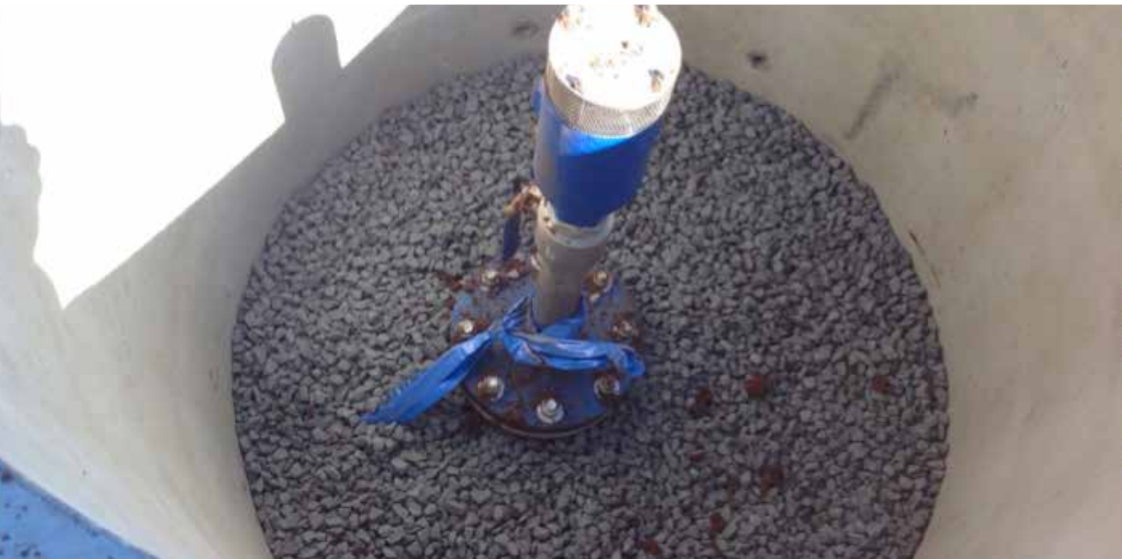
Figure 10: Completed air valve installation
