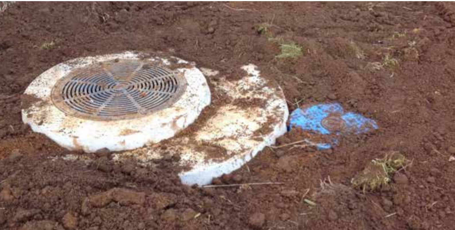
Figure 6: Scour or drain valve pit
