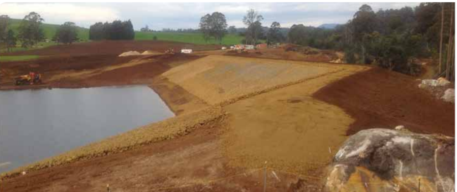
Figure 2: South Riana Dam completed earthworks
