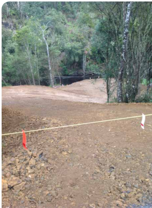
Figure 4: Blythe River pump station pad from South Riana Road
