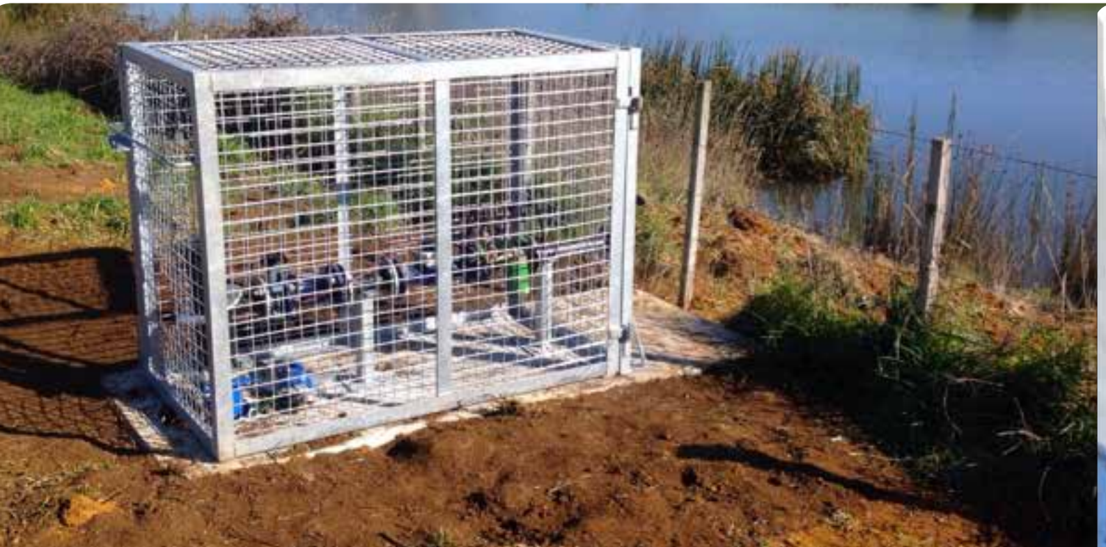
Figure 8: Completed outlet cage Cuprona
