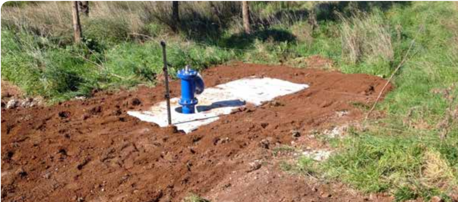
Figure 7: Outlet riser and slab waiting for valve train and cage
