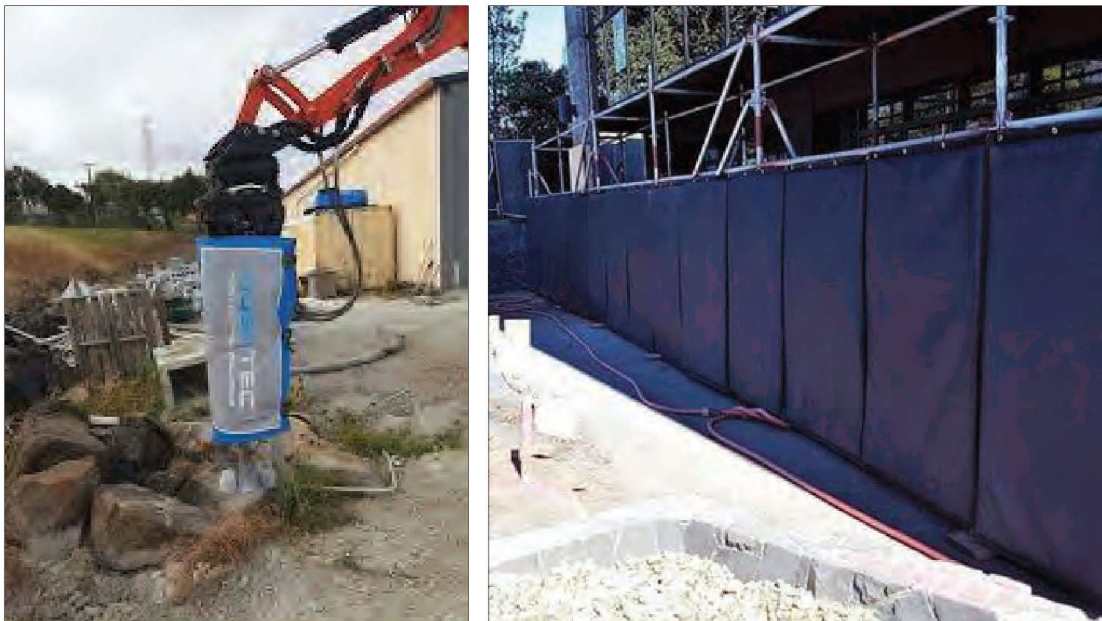
Figure 7-2: Rock breaker shroud and acoustic curtain.
