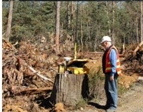
The excavators digging the pipeline channel were GPS-controlled (lower right) from a base station (lower left).
