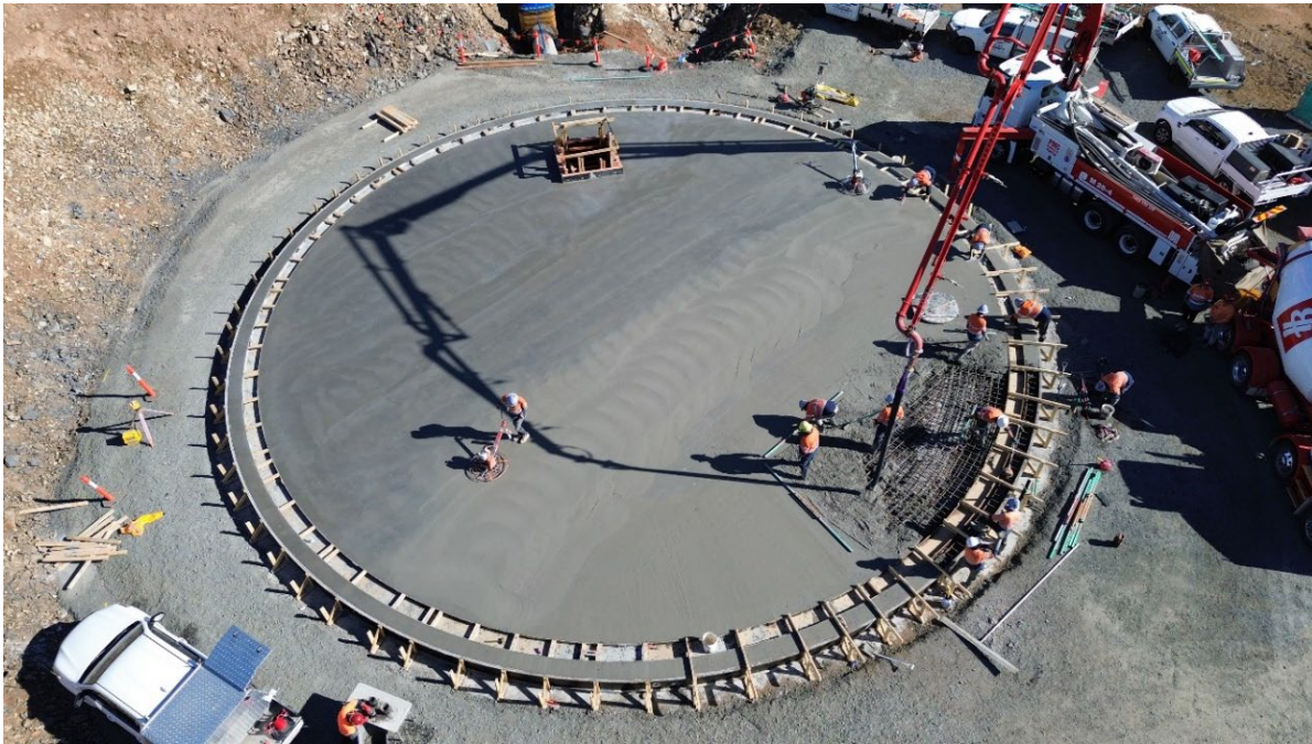
Valleyfield Balance Tank foundation being poured
