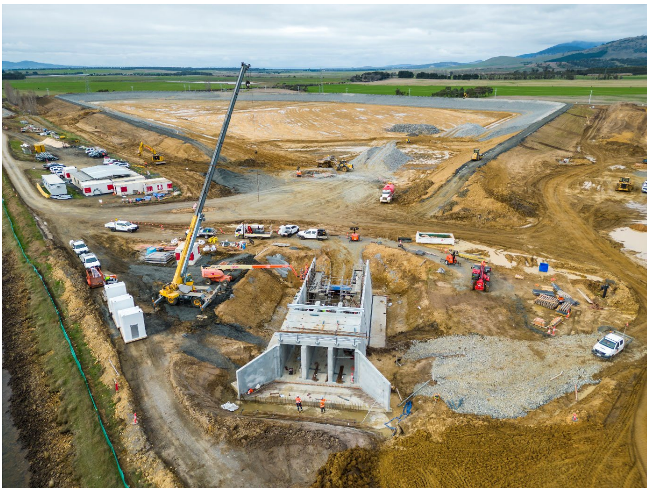
Poatina Buffer Dam and inlet structure in the foreground
