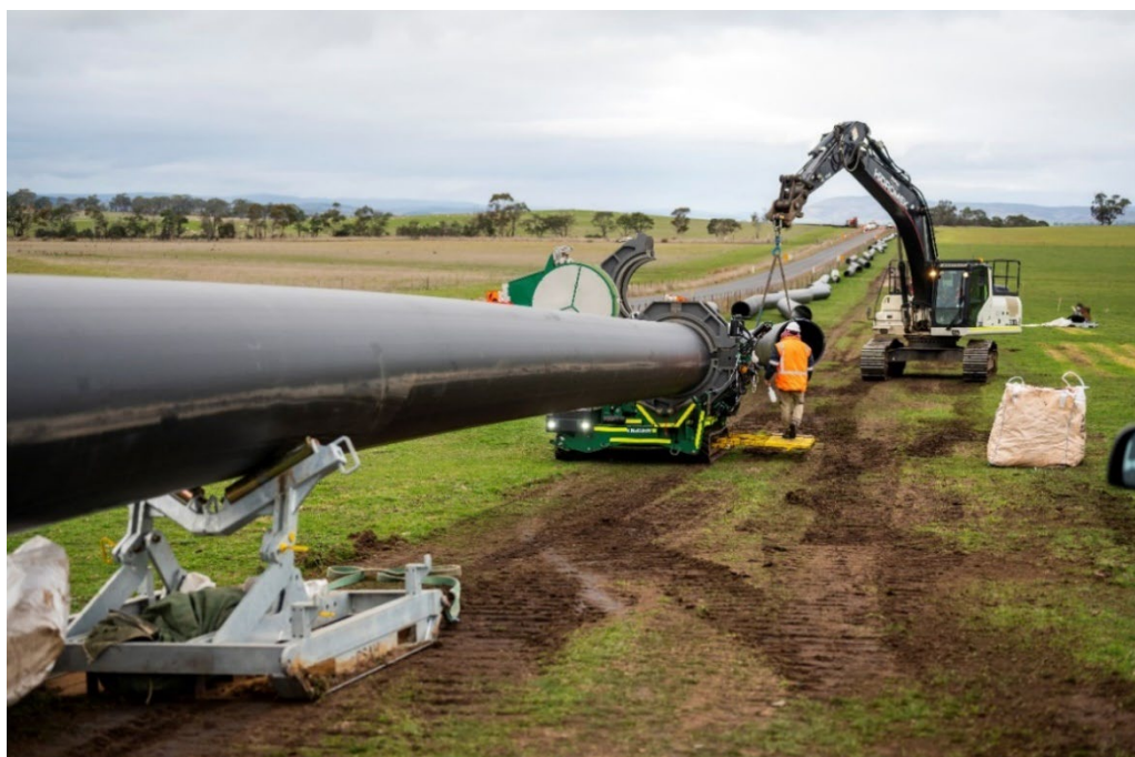
Pipe welding underway at Mt Joy Road
