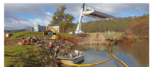
Pic: Intake screen formwork installation at Quamby
