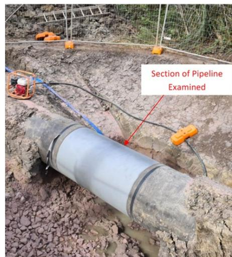
*Picture: An example of one of the pipeline sections examined after its coating was removed and the pipe was sandblasted clean ready for inspection*
